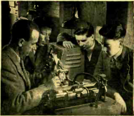
A group of young trainees being coached in the operation of a recorder cutter head.
